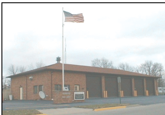
Thomas Dore Memorial Fire Station
